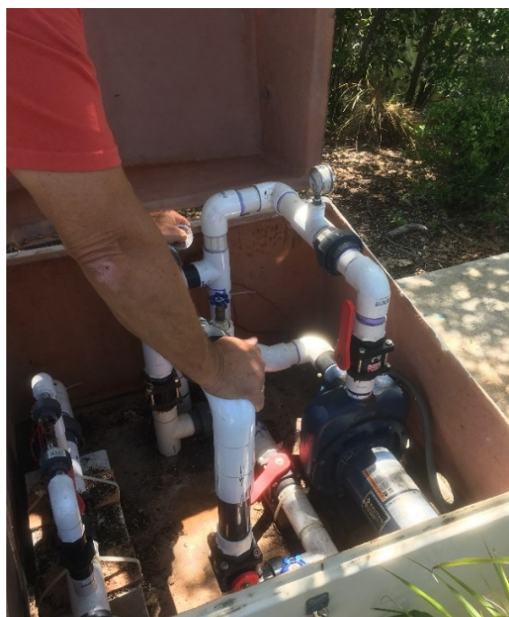
Fig. (2a and b). EMOH device connected to 1 HP pump with PVC piping. Nanobubbles at the surface, rising from near the bottom, shown in 2b. (courtesy Matt Iles and Brian Bailey). (A higher resolution / colour version of this figure is available in the electronic copy of the article).
